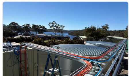
Rooftop Cable Tray Installation
