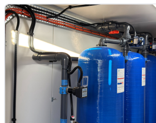
Remote Water Treatment Site
