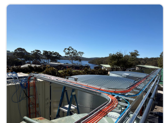
Rooftop Cable Tray Installation
